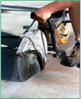
Photo showing cutting of control joint
